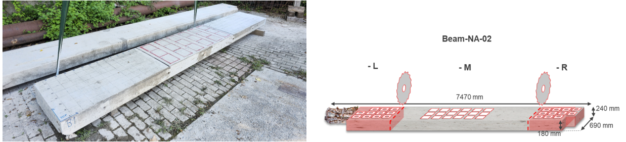
Figure 6. Extracted reinforced concrete beam with cutted edges and testing areas marked in red, from (Al-Shboul et al., 2026b)
