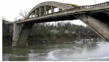
Fig. 4 An existing through-arch bridge
